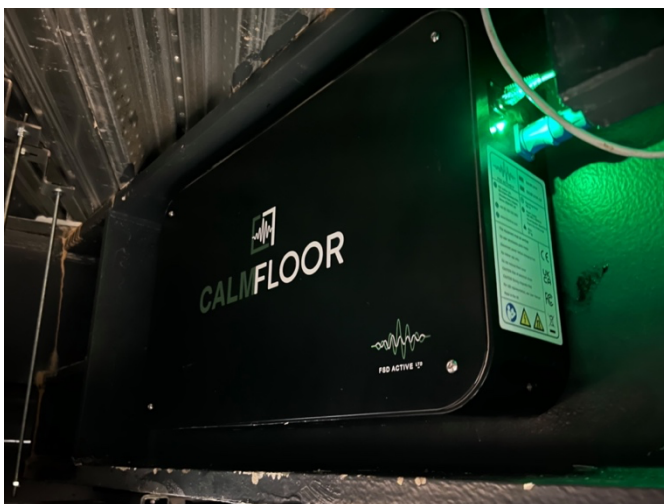
Figure 3: The alternative – the 67kg CALMFLOOR AMD attached to a steel I-beam supporting a composite steel-concrete deck. Courtesy of FSD Active Ltd.
